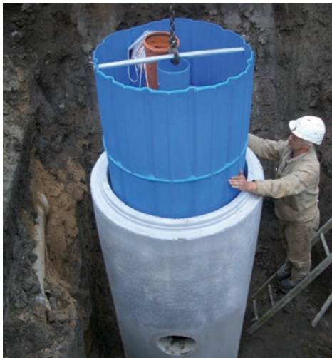
Hydrofilter 1000 monteras i befintlig 1000 brunn.
